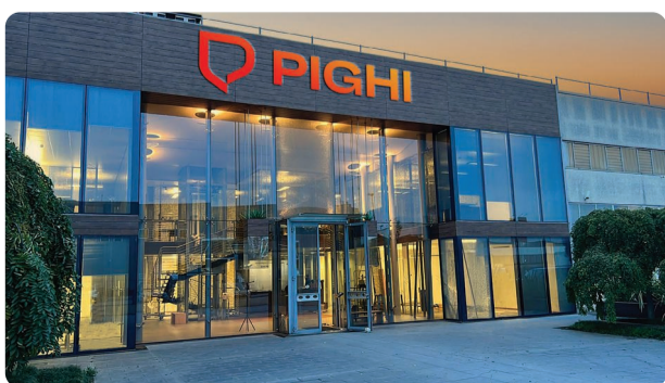
Pighi new headquarter, work in progress
